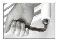
3. Fit the radiator valve, compression nut and olive over the end of the pipe, do not tighten yet. By hand turn it to the correct position and connect to the valve tail and nut fitted to the radiator, then tighten using a spanner. Repeat the same process for the lockshield valve on the opposite side.
